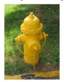
Water tankers or "tenders" are available from surrounding departments if the occasional need arises. When new hydrants are installed, they should be specified to have "Storz" fittings on the primary or steamer outlet at little or no marginal cost.
