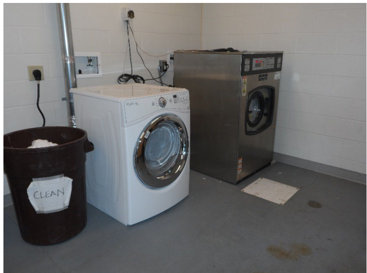
Right: A commercial extractor for cleaning turnout gear is now required in addition to the traditional washer.
