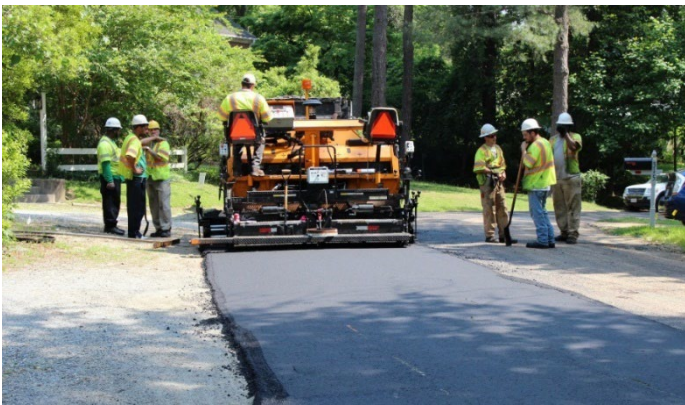
Paving Crew creating a safer York County Street
